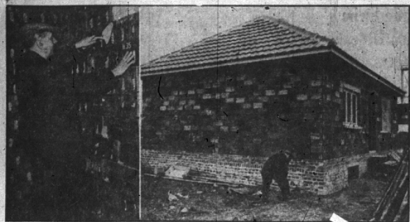
HOME FROM THE WAR —A German architect, turned homebuilder, is shown, left, putting the finishing touches to one wall of the cottage he is constructing in Frankfurt, Germany. Needs a place to live and lacking funds for conventional materials, the builder used wooden ammunition boxes that had been stacked in a former German army depot. To give the boxes the necessary strength to support the roof the compartments designed to hold shells were filled with cement. At right is a view of the outside of the building as the architect caulks basement bricks.
