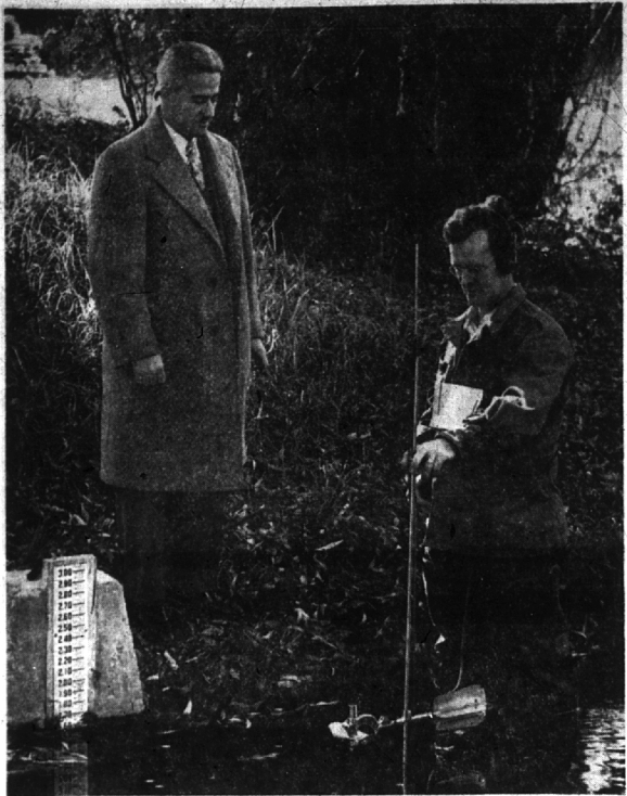
ENGINEER A. D. ASH WATCHES FIELDMAN L. G. STEARNS Current meter is used to check speed of water on Rouge (Dick Shirk Photo)
