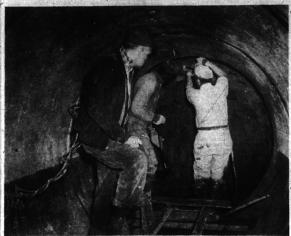
This sewer construction crew works 50 feet under the Grand Trunk railroad tracks in putting in the new Webster relief sewer which will give substantial benefits to homes on the eastern edge of the city.
