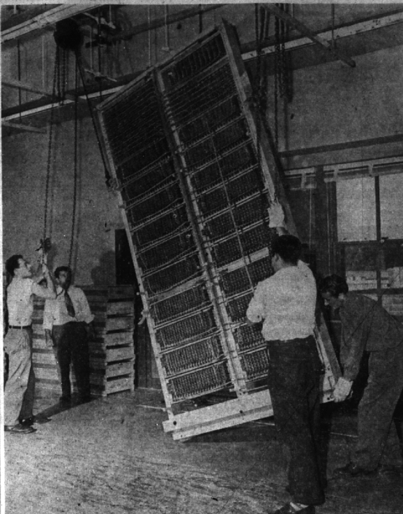
First unit of dial equipment is hoisted into place by Western Electric Co. installers on the second floor of the Michigan Bell Telephone Company's new building at 160 Martin. The new $2,225,000 dial system is expected to be ready next summer according to Walter B. Fausser, manager of the local exchange. Michigan Bell moved into its beautiful new building only a few weeks ago when its business office was opened to the public. Literally millions of hand-soldered connections must be made to link individual units of dial equipment into Birmingham's network of telephone lines.
