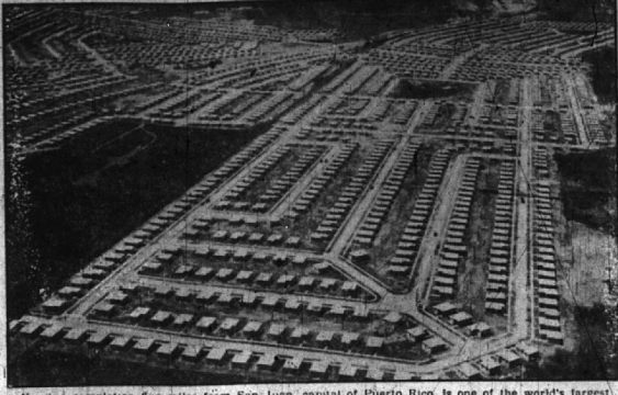
Nearing completion five miles from San Juan capital of Puerto Rico, is one of the world's largest private housing developments, Puerto Nuevo. Above are some of 3500 concrete, five-room dwellings, built in slightly more than a year's time, with 1500 others soon to be completed. They will be for an average of $4000 and were constructed by a South Carolina builder in co-operation with the FHA and Puerto Rico government to alleviate the island's acute housing shortage.
