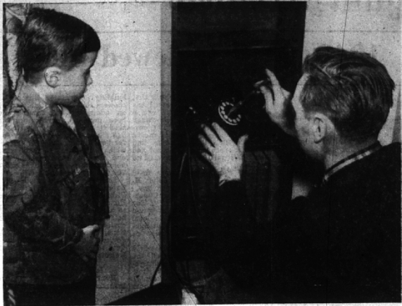
Johnny Mange, 6, intently watched as Bill Kreger, installer for the Michigan Bell office here, puts a new dial on the phone in Johnny's home. The dials were installed in March on all phones here preparatory to the automatic dial exchange cutover here in the early summer of 1950.
