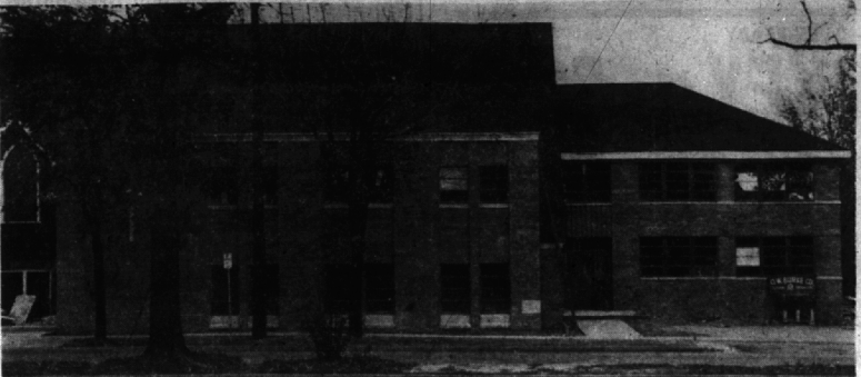
This picture of St. James Episcopal Church presents a side view of the recently completed and dedicated addition which was built at a cost of approximately $150,000. The old section is shown to the extreme left and continued from it is an enlargement of the church proper, permitting a greater seating capacity. At the far right are the ten new class rooms and meeting rooms for the various church guilds and clubs. Also included in the expansion program were new kitchen and dining facilities. The Rt. Rev. Richard S. Emrich, S. T. D., Bishop of the Episcopal Diocese of Michigan, officiated at the dedication ceremony Sunday.
