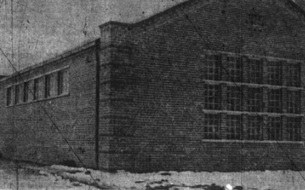
This is the home of the new Longacre-5 dial telephone exchange for West Bloomfield. It was cut into service quickly on Monday. Created from parts of the Birmingham, Pontiac, and Farmington exchanges, the newest Michigan Bell Telephone Company office was built in recognition of the growing community area of interest in the West Bloomfield area.
