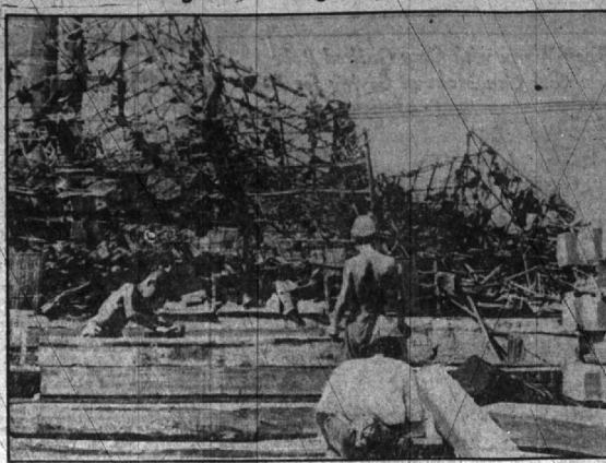
Nagasaki, second city devastated by the atomic bomb, is slowly taking shape again. Here Japanese workers prepare timber for rebuilding homes. This area is about half a mile from the center of the blast. Twisted steel in background indicates its terrific force. (Signal Corps photo.)
