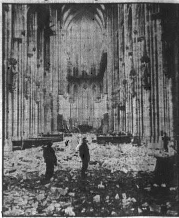
American soldiers survey damage in famed Cologne Cathedral—a litter of masonry from upper regions of the edifice. The Gothic pillars appear undamaged.
