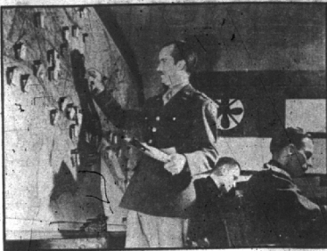
This is the flight control room at La Guardia Field, N. Y., where the course of every flight in that area—hundreds daily—is followed on a map, a marker moving magnetically along the plane's course according to the speed of the plane. Knowing at every moment exactly where each aircraft is helps to avoid accidents. Maj. Raymond S. Talbot of Hampton, Va., is shown at the map. Seated, left to right, are Lieut. John S. Thome of Covington, Ky., and Elmer J. Schmalz of Minneapolis, Minn., who gather information on weather, traffic, and field conditions.
