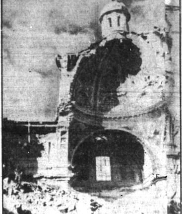
This shows a job done by the fleeing Germans on the 100-year-old St. Thomas Cathedral in Ortona, Italy, after the Canadians entered the town. Destruction of the church was one of the enemy's last acts, an attempt to impede the advancing Allies. (OWW radiophoto.)
