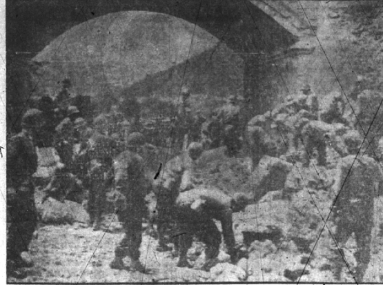
Near Utri, Italy, American engineers clear the blasted Applan Way where it passes beneath a railroad viaduct. This forerunner of the modern super-highway was begun in 312 B. C. by Appian Claudius Caelus the Censor. Succeeding emperors extended it until it terminated at Brundisium (Brindisi) near the Adriatic coast about 243 B. C., furnishing a trade route to the east. Originally it was a two-lane, stone-surfaced highway 49.5 feet wide, 412 miles long. (Army Radio-Teletype.)
