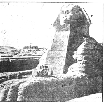
SPHINX WEARS CHIN STRAP—A wall and sandbars have been erected to protect the Sphinx from possible damage.
