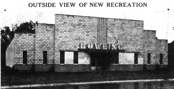
Photographer Al Arnold had to set up his camera in his car to take this picture of the new Birmingham Recreation during the all-day rain on Tuesday. The building is 75 feet wide and extends back 135 feet to Brownell street. A new type of cement brick was used in the construction plus liberal use of glass brick around the front doors. The "Bowling" sign is in neon.
