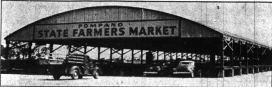
Massive structure above is the world's largest produce exchange under one roof. This new Farmers' State Market in Pompano, Fla., is 1000 feet long and 98 feet wide.
