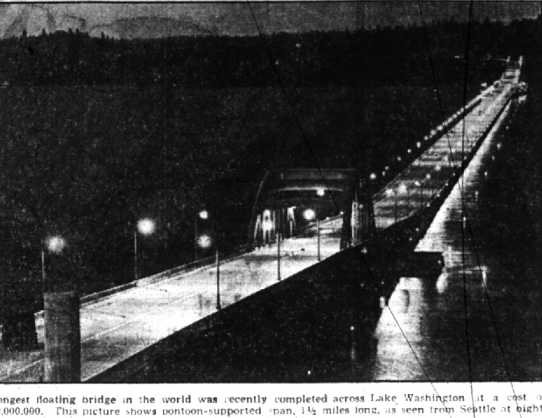
Longest floating bridge in the world was recently completed across Lake Washington at a cost of $2,000,000. This picture shows pontoon-supported span, 1 1/4 miles long, as seen from Seattle at night.
