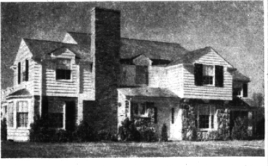
Mrs. Lida Limbocker, of Detroit, her son, Harry, and two daughters, Eleanor and Jane, have just taken up residence in their new home at 1069 Brookwood Court. Walter Baulin, well known local architect, did the designing and Ralph H. Scheel, the general contractor. Snyder, Buck & Bennett, brokers, effected the property transfer.
