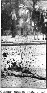
Gushing through State street, Chicago, this baby geyser is one of several that burst from cracks in pavement as compressed air pushed through supporting clay on roof of city subway, now being dug.
