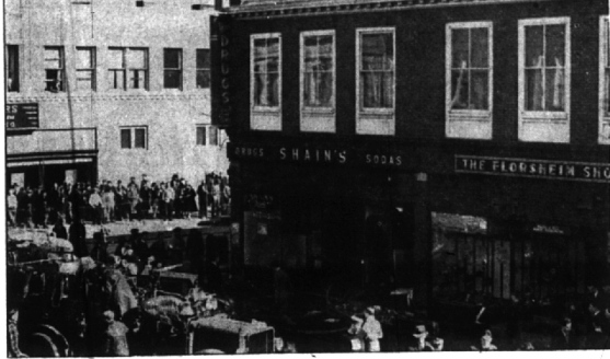
Streets were roped off in the business district Tuesday, while firemen worked to check the blaze in Shain's Drug Store. West Maple and Pierce street, which threatened the entire block and caused damage estimated at $5,000.
