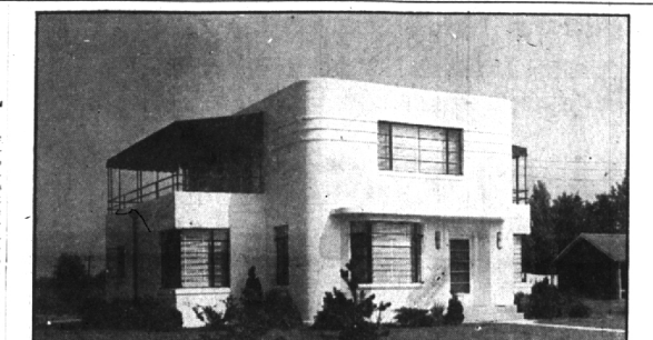
A rather unusual use of concrete blocks for the exterior walls of this modern house is shown above. Note the rounded corners and the slight projection of the masonry at the head of the second floor windows. The concrete walls have been painted white. Steve Jekel, Architect.
