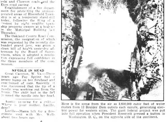
Here is the scene from the air as 3,600,000 cubic feet of water rushes from 12 Boulder Dam outlets each minute, generating electric power for western cities. The giant federal project was put into full operation when President Roosevelt pressed a button in Washington, D. C., on the opposite side of the continent.
