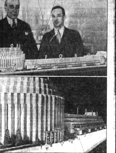
Henry Ford and Edsel B. Ford show to Rufus C. Dawes (center), president of the World's Fair, the scale model of the giant Ford Exposition building to be built at the 1934 Fair, (Lower) The Ford building as it will be seen from Lake Erie drive. Opposite the building is a huge park bordering Lake Michigan.
