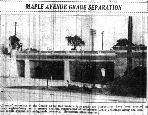
Lives of motorists at the Grand Trunk right-of-way as it crosses East Maple avenue are safeguarded by this modern type grade separation...
