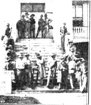
State troops standing guard on the steps of Carter county courthouse, Elizabethton, Tenn., following an attempt of textile workers to storm the building after the arrest of 250 striking employees of the American Bemberg and Glanzstoff plants. The men were arrested for picketing the roads leading to the mills.
