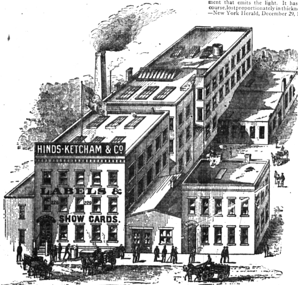
The first commercial lighting installation on land in the United States in the lithograph plant of the Hines Ketcham & Company, New York. This installation consisted of 60 lamps and one dynamo.
