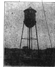
Water Tower, serving exclusively the more than 500 acres of Bloomfield Village. Good water is now being pumped from a large well, having a capacity of 700 gallons per minute—over a million gallons a day. This is half as much water as that used by the entire city of Royal Oak. A water main will be in front of every Bloomfield Village lot within 30 days.
