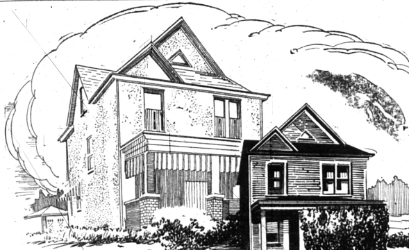
"P-Two-Fourteen" Steel Fabric Reinforced Stucco "overcoat" applied to a frame dwelling at Moonessen, Pa.
