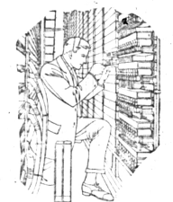
Maintenance Man Working on Switchboard Adjustment
