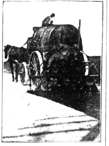
Surface treatment of Macadam Road with Bituminous Material and Stone Chips.
