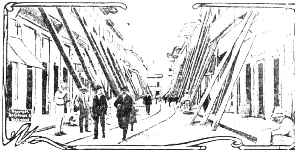
Buildings in Mexico City propped up by timbers after an earthquake. The street proper is propped up by a wall of timbers, and the buildings are supported by a wall of timbers.
