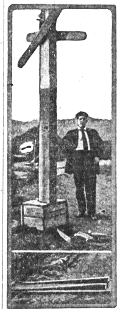
Highway Block Signal and the Trap at the End of the Dangerous Stretch Which Operates It.
