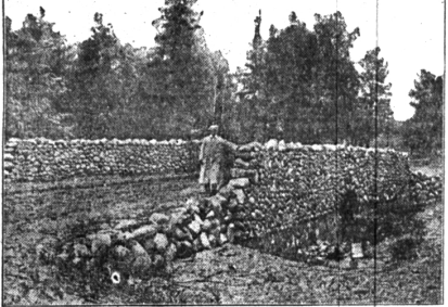
Stone Bridge on West Michigan Pike in Leelanau County.
