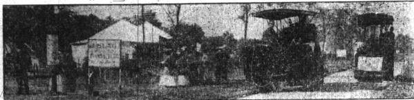
Building Good Roads at the Michigan State Fair. This Work is done under the Direction of Experts and is a Great Educational Feature.
