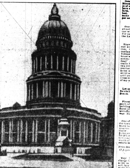
This Structure, Built at a Cost of $7,000,000 Was Wrecked by the Earthquake and Flames Committed the Destruction.
