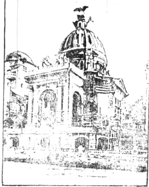
PHOTOGRAPH MADE BY THE AMERICAN PAVILION.
