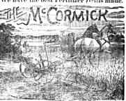
You have run a mower perchance since boyhood, but you never rode one of so light draft, so easy to manage, and such a powerful cutter as this No. 4 Steel Mower. Do I know what I am talking about! I do. The dynamometer power proves our superiority for light draft. It takes but a moment to grasp the lever and raise the bar. Howeasy it is done. Its long pitman gives it a powerful stroke and the guards are cleared without backing the nachine!
